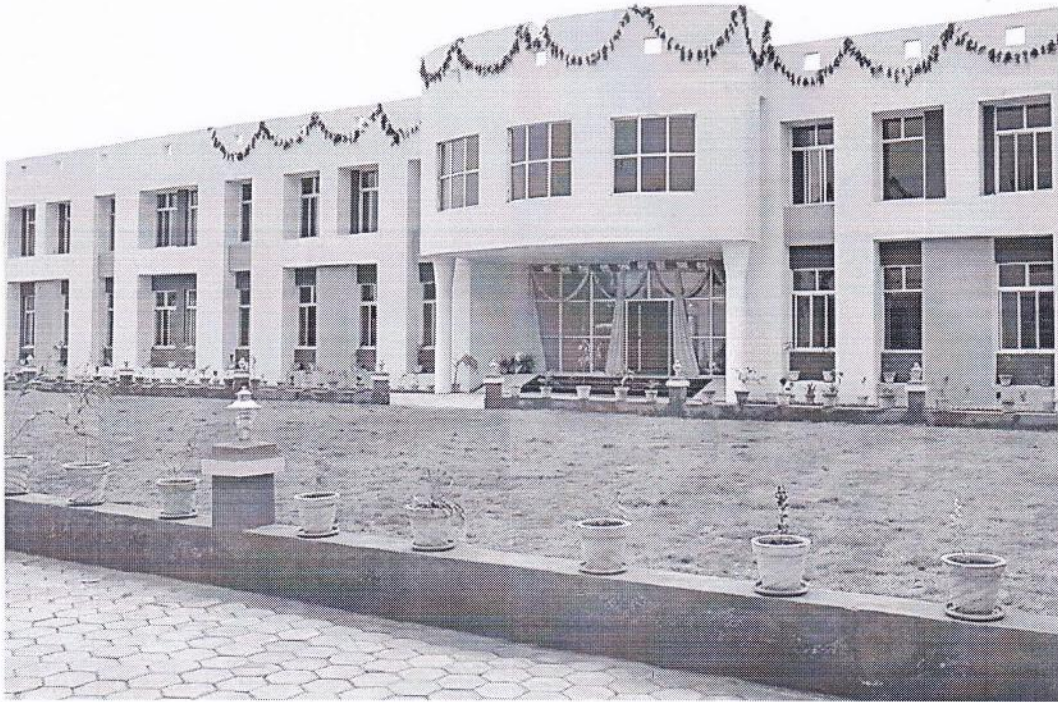
Rear view of the building
